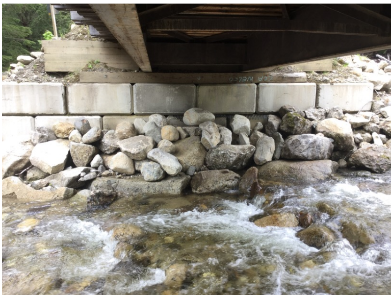
Right Bank Abutment when facing downstream
