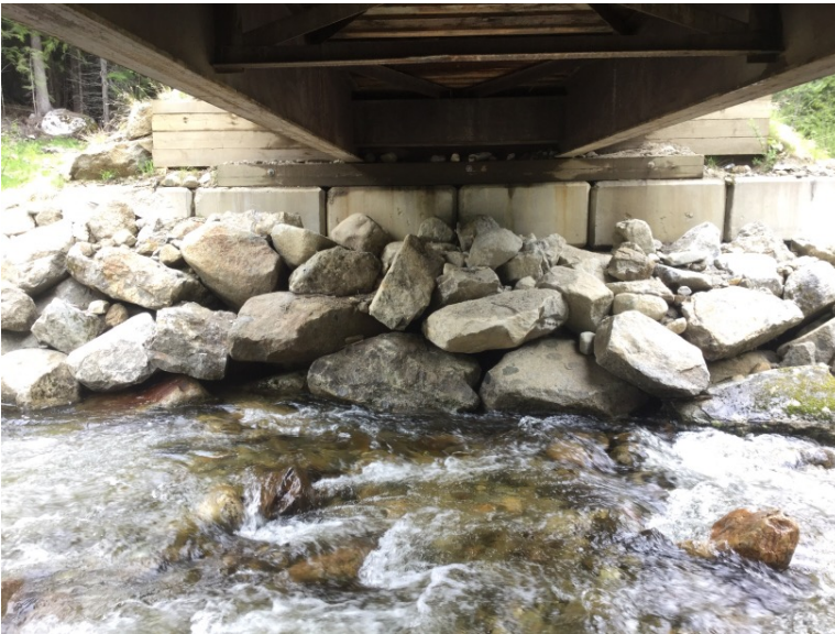
Left Bank Abutment when facing downstream
